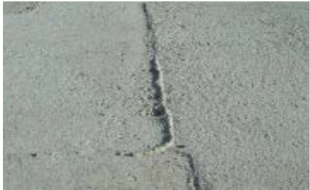
In situ concrete
